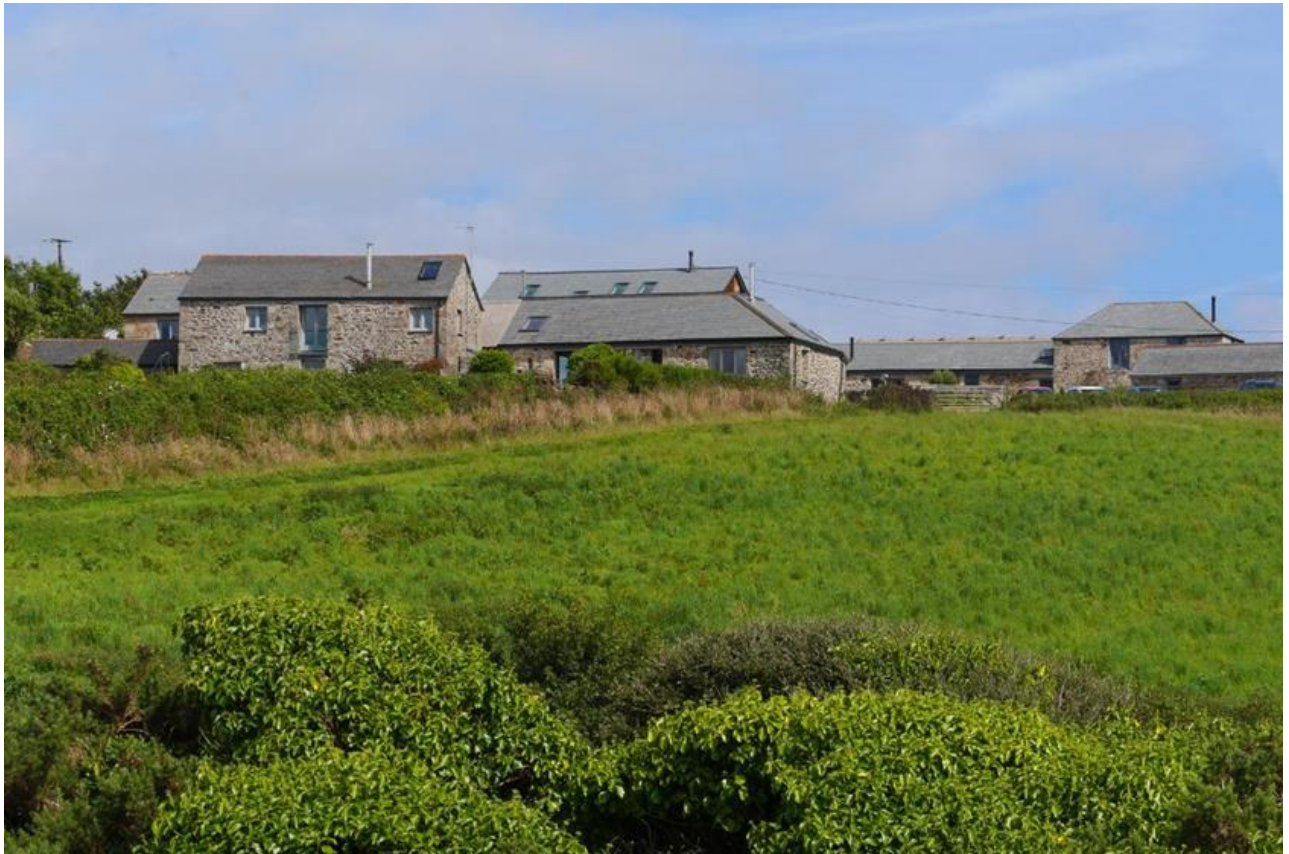
Looking south-east up to the historic farm buildings at Trebarvah
