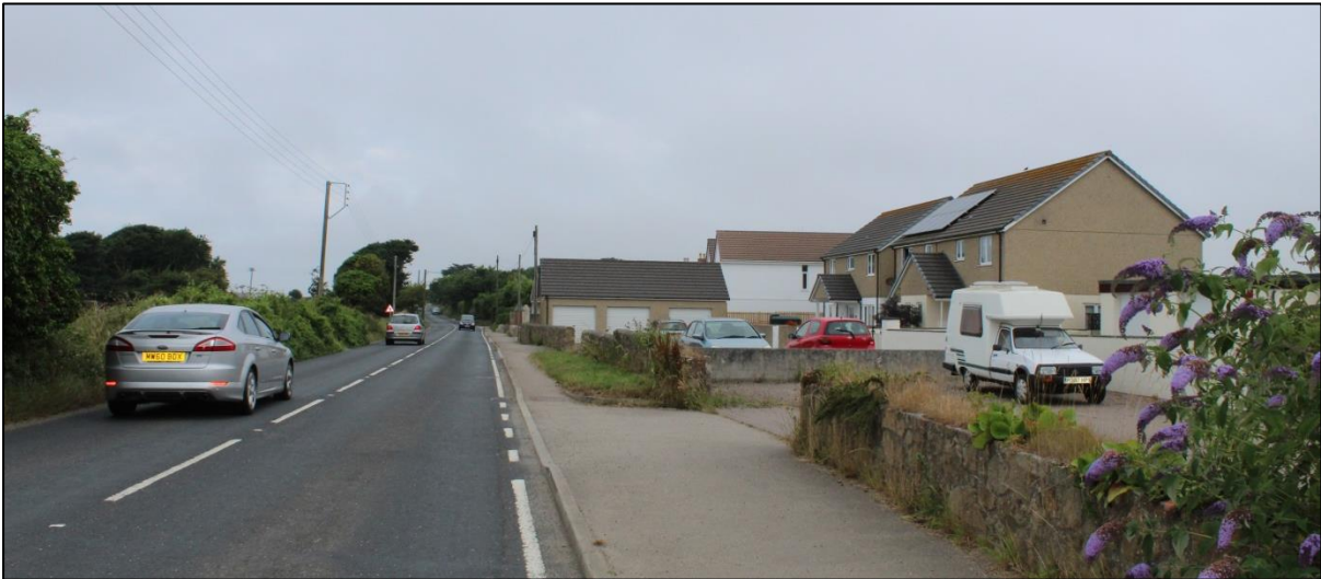
Looking west along the southern settlement boundary with the A394
